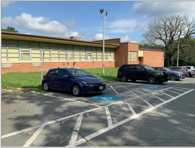
OVERVIEW OF ACCESSIBLE PARKING AREA
